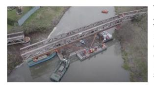
The mid-section of Berry Hill Footbridge across the Jubilee River in Taplow was removed in December. The structure has been closed to the public since May 2021 after suffering unforeseen structural deterioration. Work has been ongoing to finalise the design and start the prefabrication of the replacement bridge section. The Council's contractor is currently seeking design/programme approvals from the Environment Agency (EA). Early indications from the
